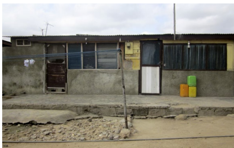
A typical dwelling in Ashaiman (Photo: R. Ayibor).
